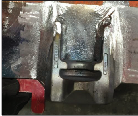
Figure 34 Inspection of Boss corner fillet weld
