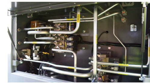
Steel pipework for better heat dissipation
